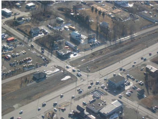
Figure 8-3: View of the intersection of the Parks Highway, the Knik-Goose Bay Road and the Alaska Railroad.
